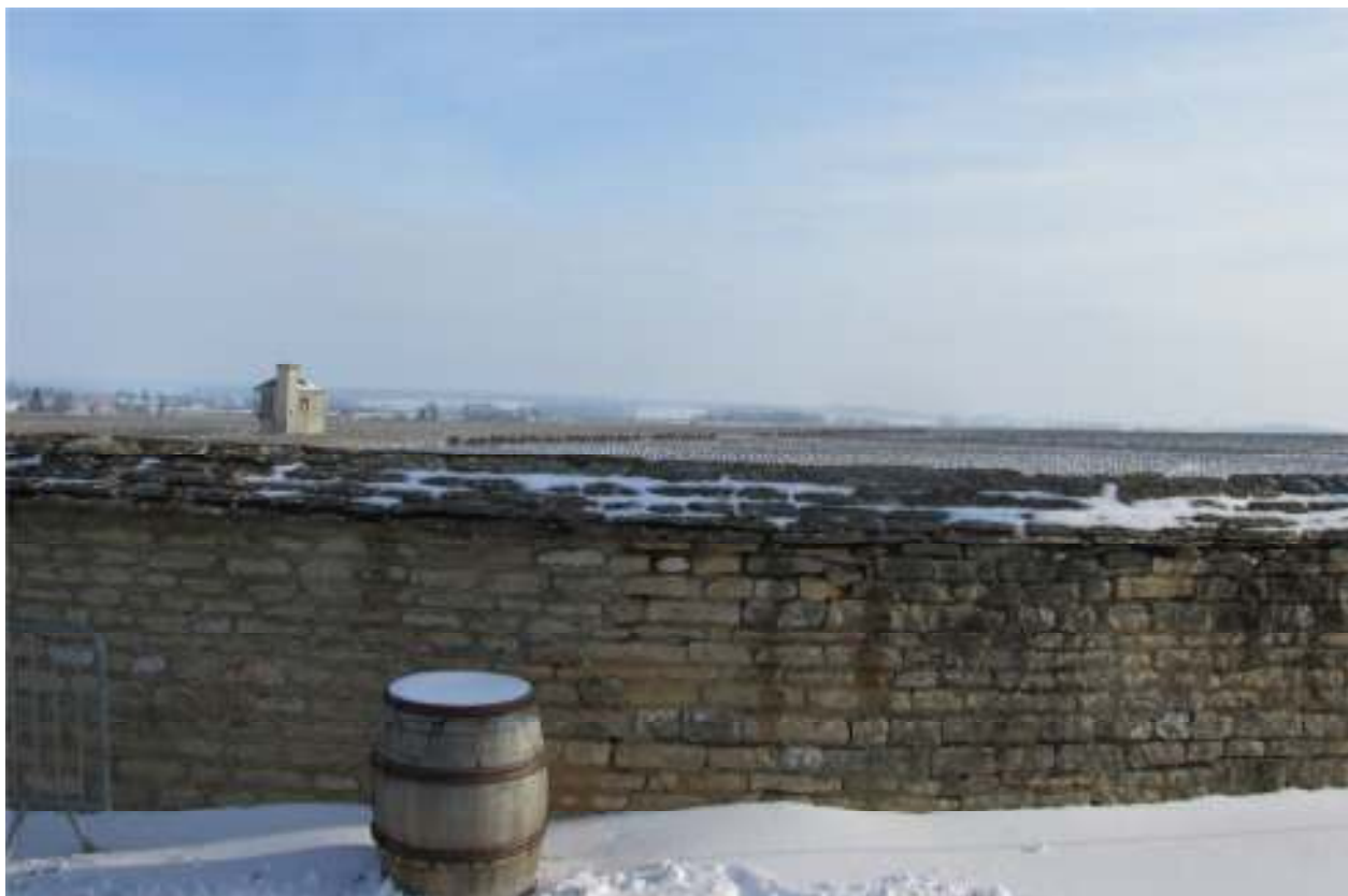
March 1 st 2018 at the wall of the Clos de Vougeot.
